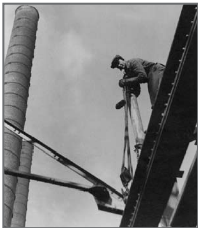
Štefan Jelovčan, monter in varilec v železarni (Štefi Muhar)
